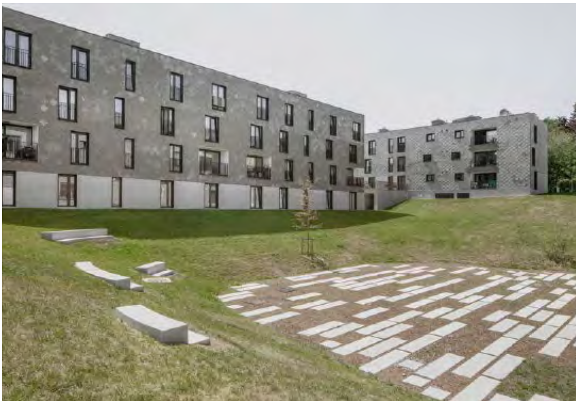
28 | Pogled na skupni zunanji prostor (vir: https://www.archdaily.com/953938/social-housing-klein-rijssel-abscis-architecten-plus , dostopano: november 2025)
